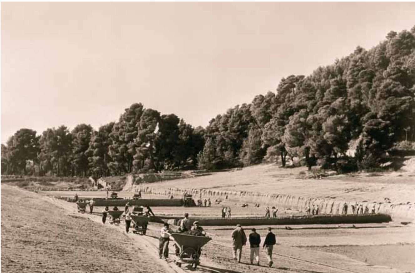
Excavation work at the stadium of Olympia, 1958 [German Archaeological Institute]
