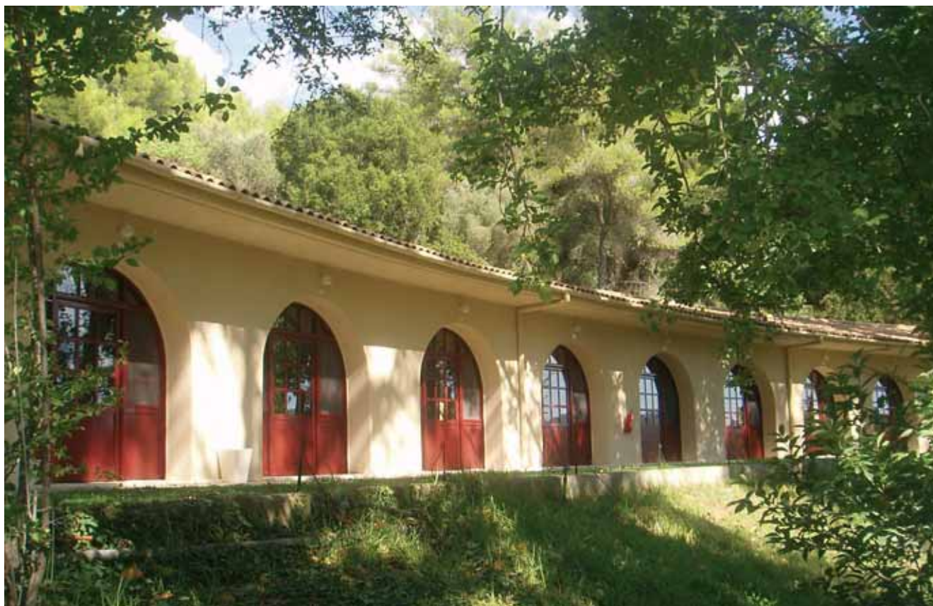
Part of the residence units in the fourth tier [photograph: Vassiliki Tzachrista, 2006]
