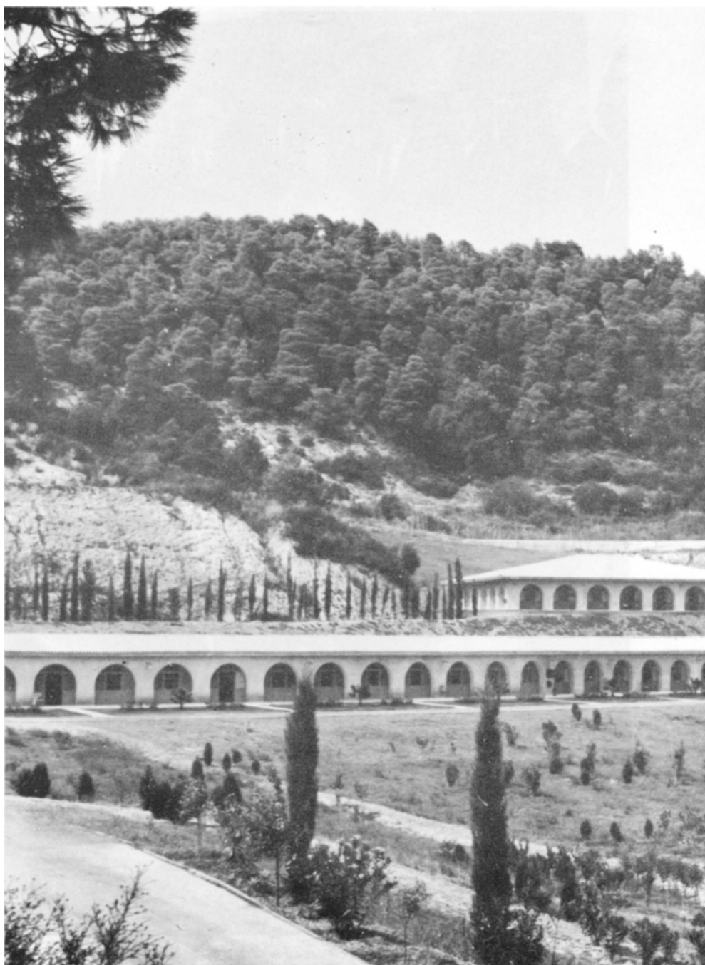
General view of the LO.A. installations in Ancient Olympia. Above: The administration offices and
