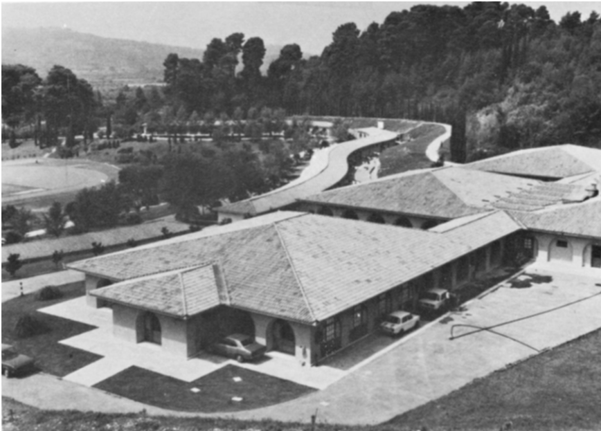
A view of the I.O.A. facilities. On the lower level, the dormitories. On the upper level, the conference hall, the restaurant, the recreation room, the offices and the library in the rear.
